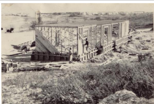
Harry Male Scout Lodge Under Construction
